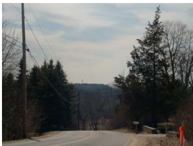
Picture Limited visibility of extremely sharp turn on Pudding Hill Rd makes a dangerous situation
