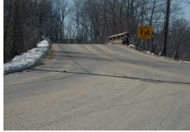
View west of limited sight distance and dangerous intersection at the Perkins Bridge/ Evans Road-Perkins Road split
